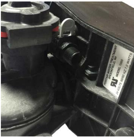
Img 8 - Brine Fitting
